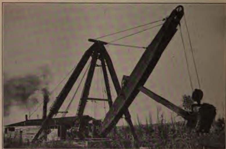
Dipper Dredge with Bank Spuds Excavating Drainage Ditch. Figure 87.
